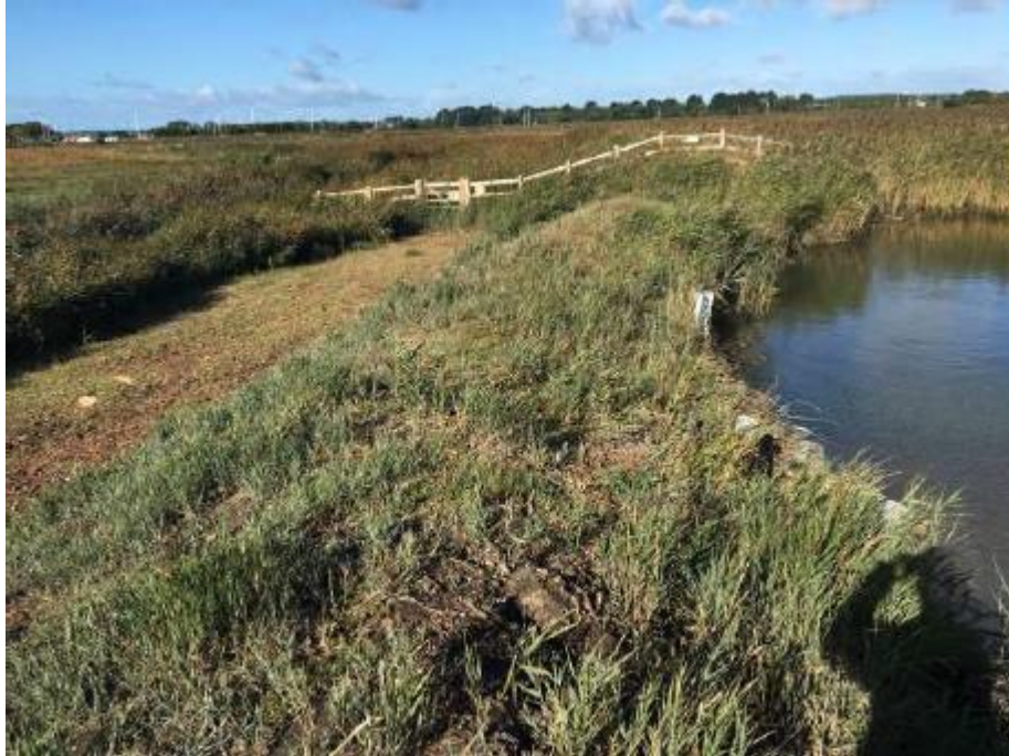
View of current Turners Cove Outfall
